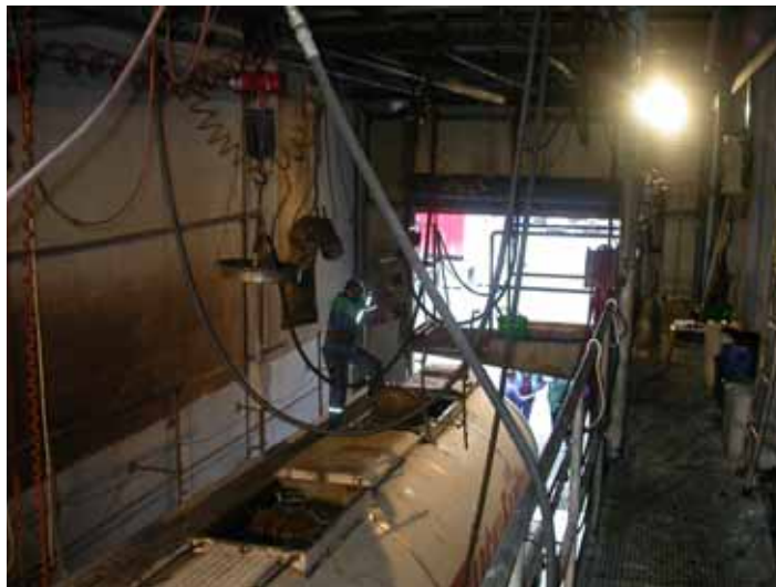
(fig.1: lowering of cleaning tools)
